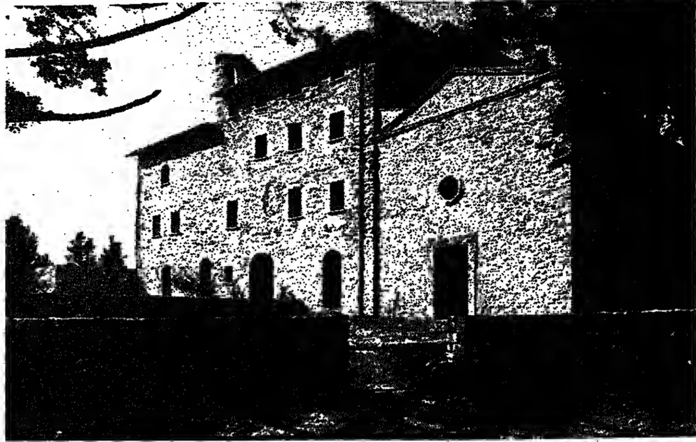
The main house at Borgo Bastia Creti, which is being converted into apartments of two to four bedrooms
